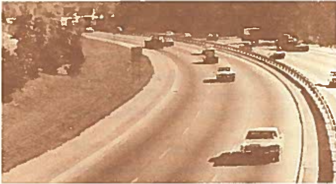
Level of Service A: Free flowing traffic, with no restriction on maneuverability and drivers able to maintain their desired speeds with little or no delay.
