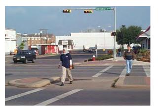
Pedestrian oriented design features: Pedestrian Refuge at median Timed Pedestrian crosswalk signalization 11-6" wide shaded sidewalks
