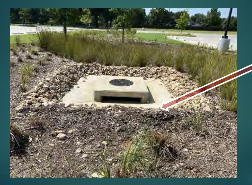
Mulch and soil washed out during rains
