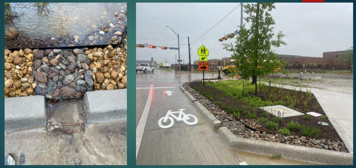
Curb cuts (18" wide) allow storm water from street to enter the swale
