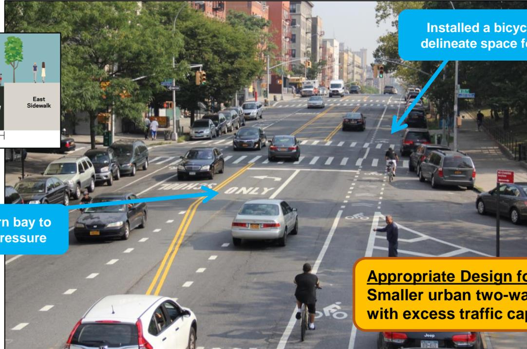
Installed a left turn bay to eliminate back pressure
