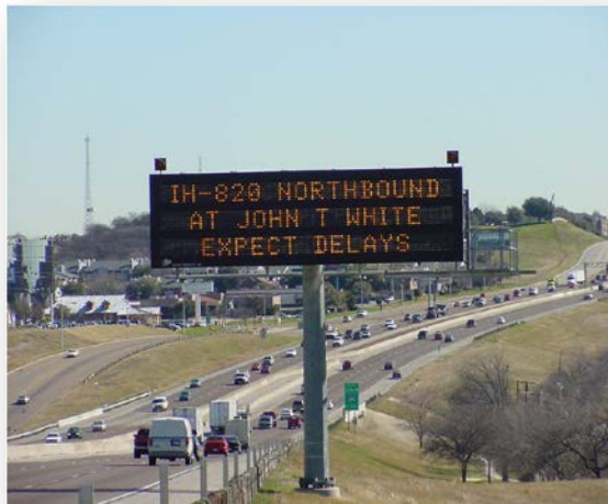
Dynamic Message Sign provides travel-time estimates and other information to improve commutes.
