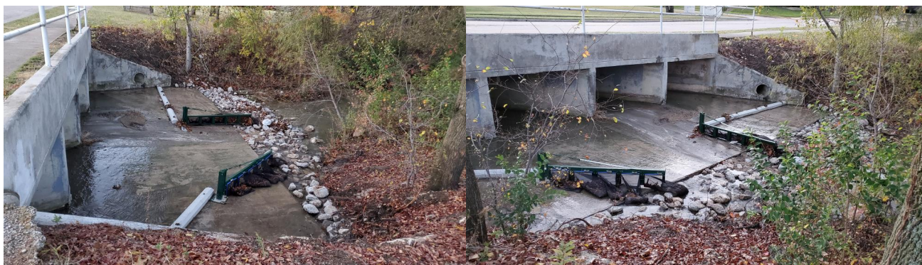
Low-Flow Open Gate with Debris in Bags
