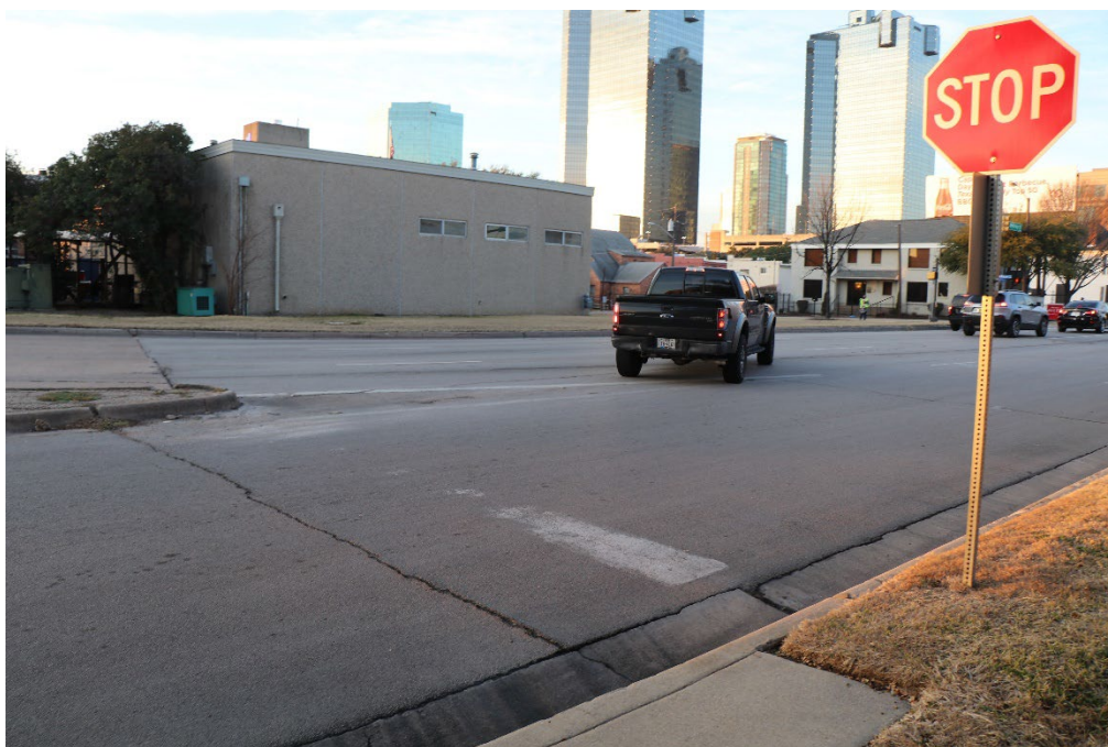
Figure 9: The City should verify whether drivers are routinely completing prohibited turn; if so, consider adding flexible vertical delineators and/or double white line to correspond with existing R4-3bT sign
