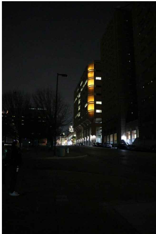
Figure 24: Non-operational City street luminaires near TCC
