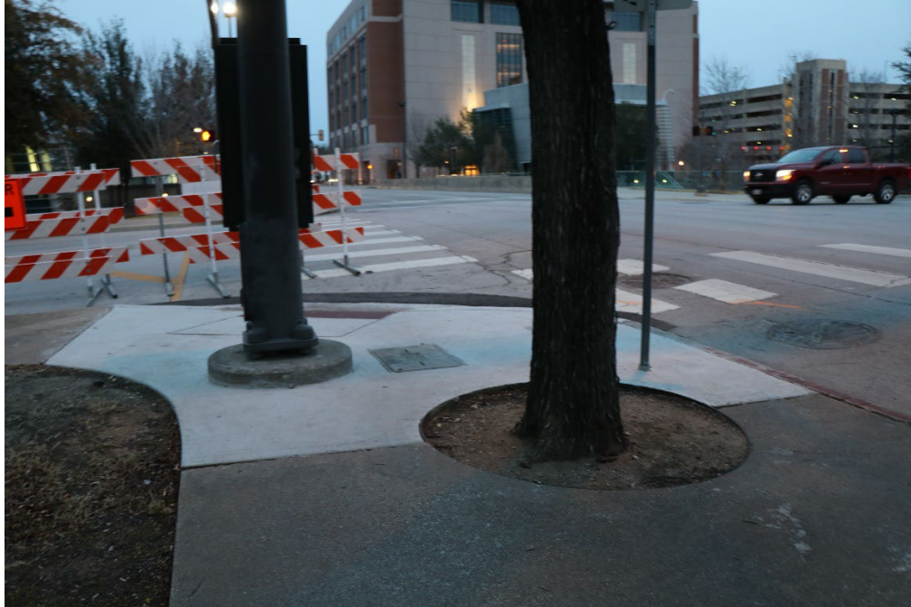
Figure 13: Obstructed sidewalks at Commerce Street
