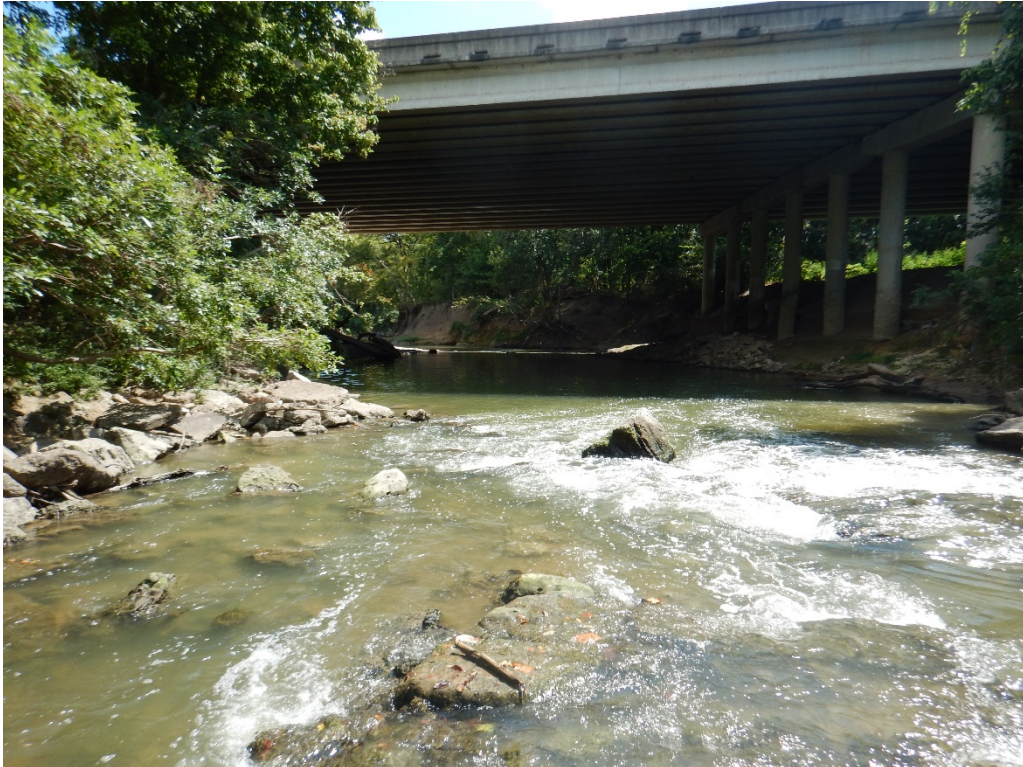
Rowlett Creek in Garland on September 16, 2021. Photo faces downstream from habitat transect 6 at a riffle with the Highway 78 bridge in the background.
