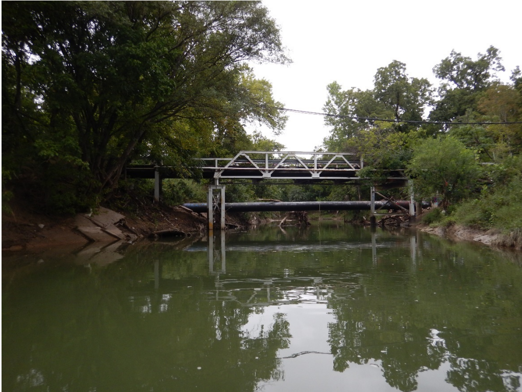
Rowlett Creek in Garland on September 24, 2020. Photo faces upstream from habitat transect 1 and shows the old Ben Davis Road bridge crossing.
