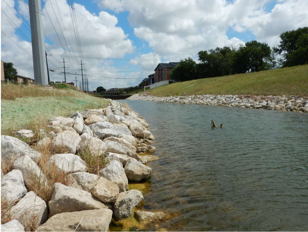
Estelle Creek in Irving on June 19, 2020. Photo faces upstream from habitat transect 5 and illustrates the engineered portions of the stream with riprap lined banks.
