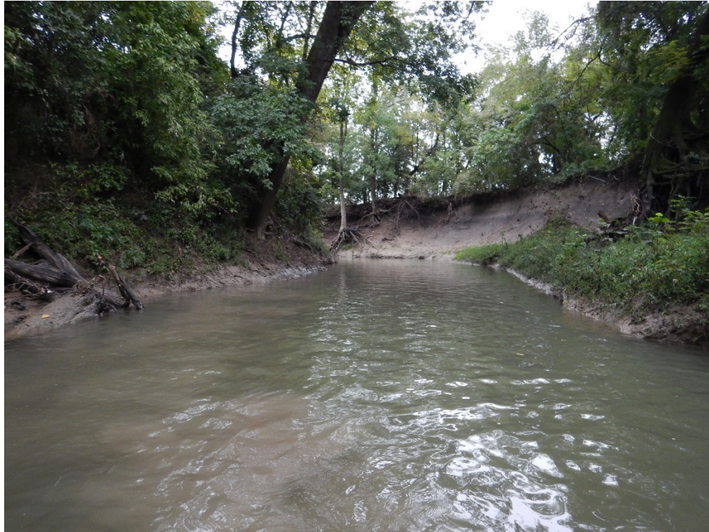
Rowlett Creek - Brown Branch in Plano on September 23, 2020. Photo faces upstream from habitat transect 1 and illustrates extensive erosion along the left bank in the background.
