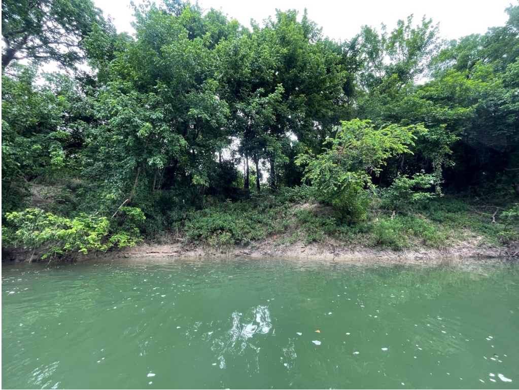
Rowlett Creek in Garland on June 23, 2021. Photo faces north to left bank at habitat transect 5. Example of high vegetative cover, low erosion potential and low bank angle.
