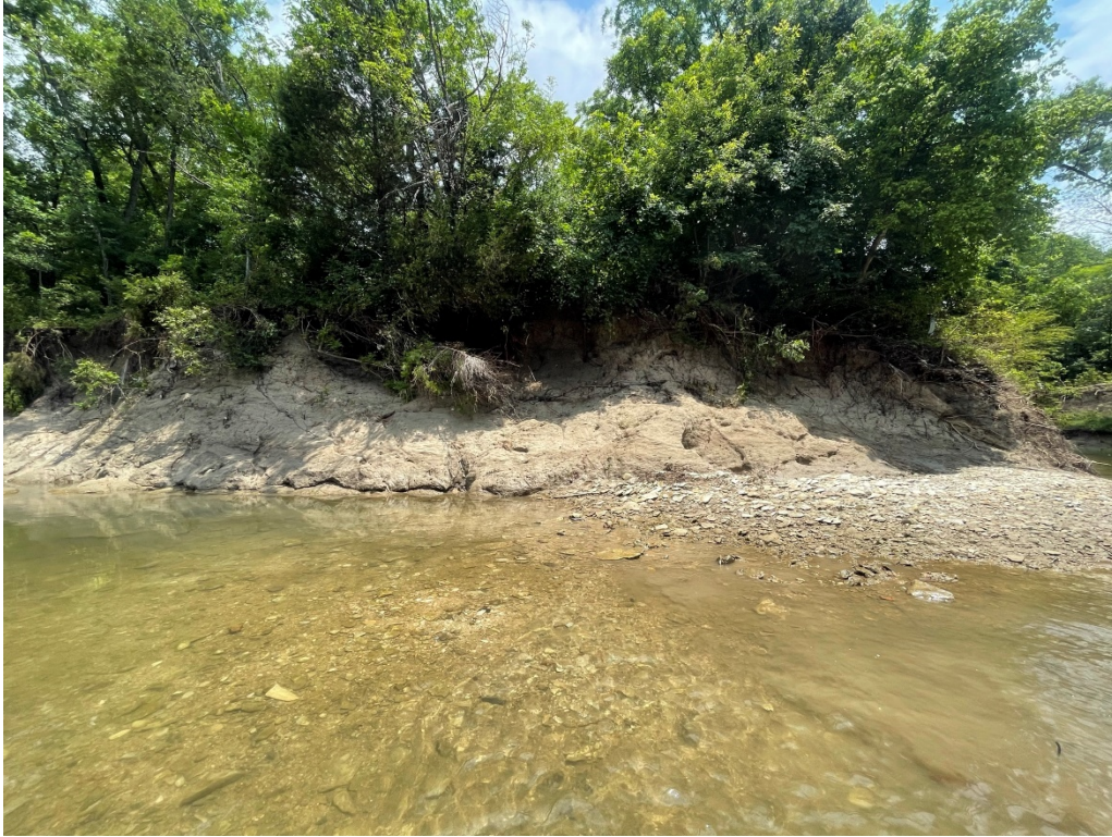
Rowlett Creek in Garland on June 23, 2021. Photo faces north toward the left bank at habitat transect 4. High erosion potential and incised bank illustrated.
