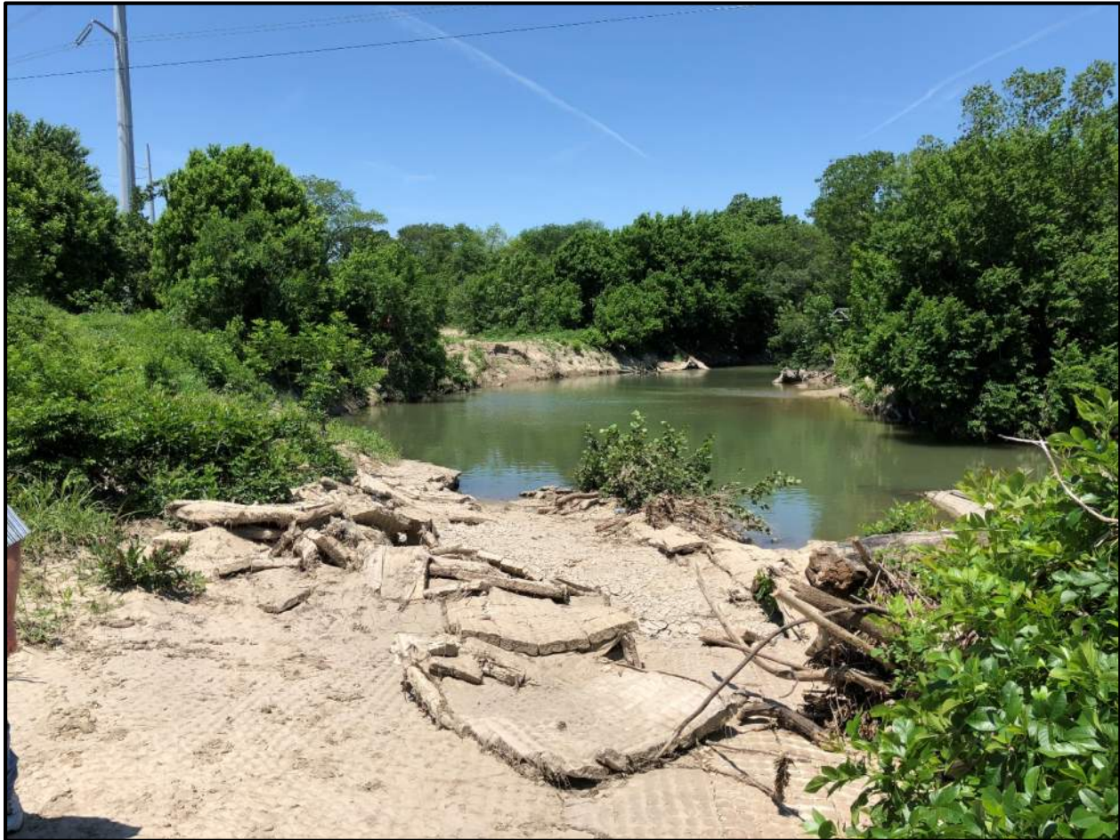
Figure 3-2: Rowlett Creek Downstream of the Atchison Topeka and Santa Fe Railroad Bridge on May 10, 2018. View is upstream towards Atchison Topeka and Santa Fe Railroad bridge. Photograph taken from the south shore (right bank).
