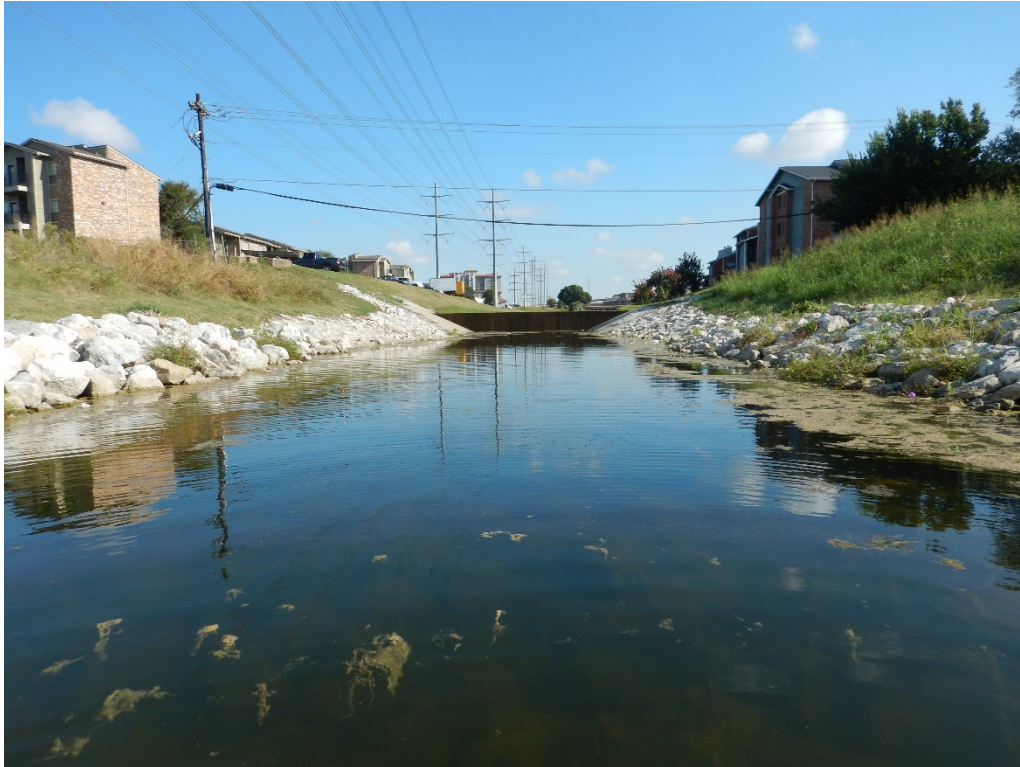
Estelle Creek in Irving on September 17, 2021. Photo faces upstream from habitat transect 2, illustrating the riprap lined banks and dam structure in the background.
