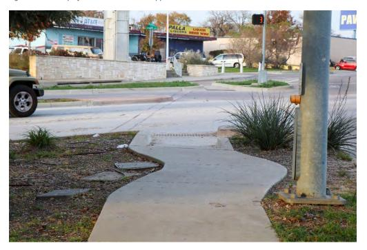
Figure 21: Several of the push buttons were placed away from the crossing point and had incorrect arrows on the plaques.
