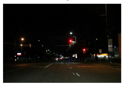
Figure 5: Meadow intersection at night, with missing street name sign on the westbound approach. The addition of the retroreflective background around the signal helps with visibility of the signal indications.
