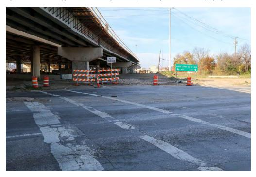
Figure 11: Stop bar and crosswalk markings that should be removed as they are no longer applicable.
