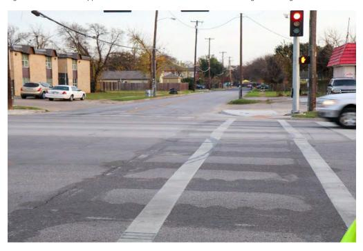
Figure 19: Crosswalk at Holmes, showing removed ladder style markings, and tire marks from cars doing "donuts."
