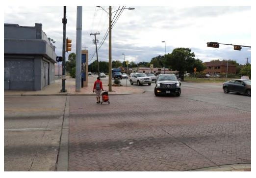
Figure 7: the sidewalks and crosswalk ramps along MLK don't line up, requiring out of direction travel for some users, along with push buttons in improper locations.
