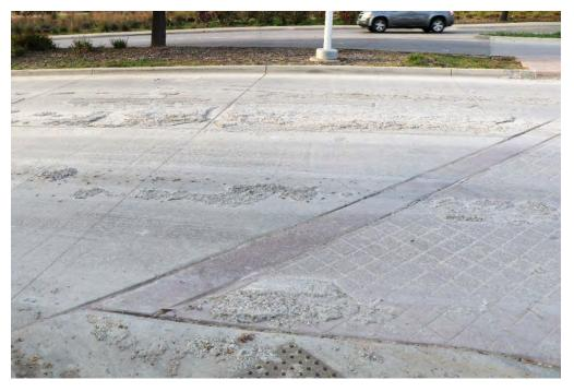
Figure 20: Build-up of Debris on the Forest approach to MLK.
