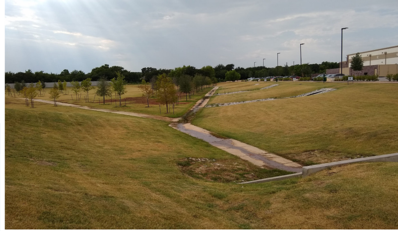
Multi-Purpose Detention Area in Denton, TX. (Source: Tetra Tech)
