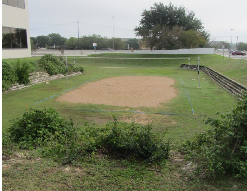
Organic Filter in Austin, TX. (Source: courtesy Troy Dorman)
