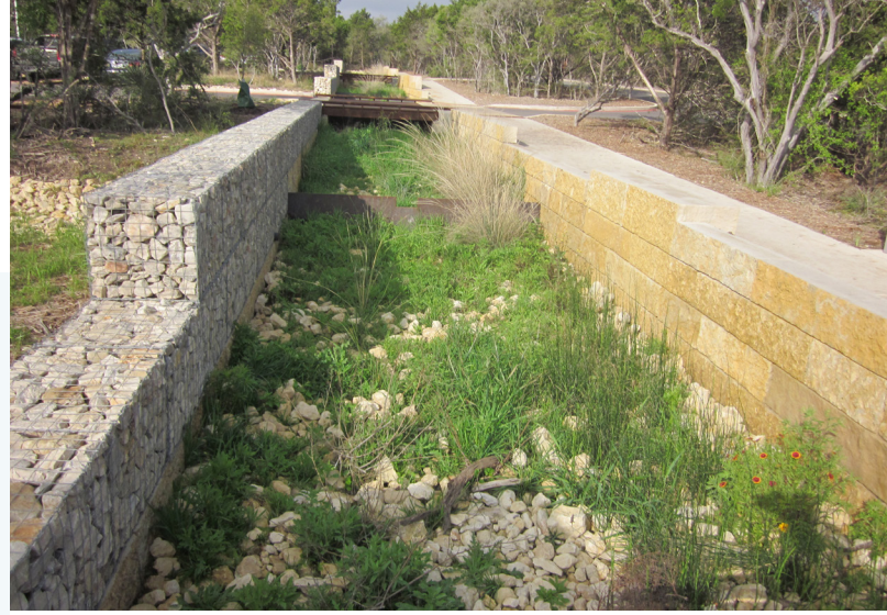
Open Conveyance Channel in Herdberger Park, San Antonio, TX. (Source: Tetra Tech)
