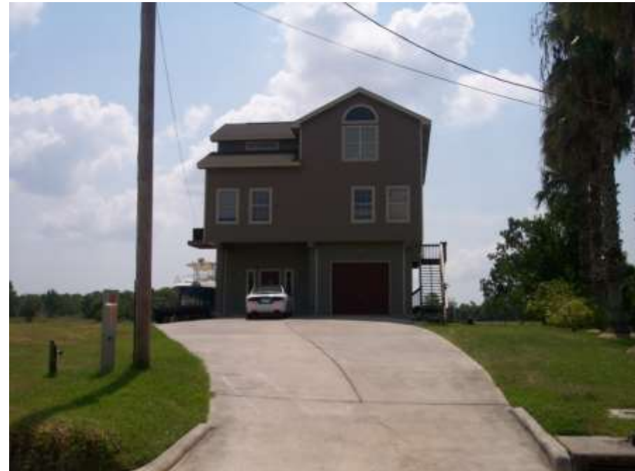
House in floodplain with habitable space below the BFE
